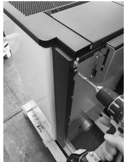
Fig. 37 - Fix the complete side panel
