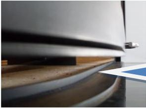
The air flow entering the fireplace is accelerated by the reduced passage under the door. This air causes the fire to be over active. The wood burns too quickly The appliance becomes less efficient.
